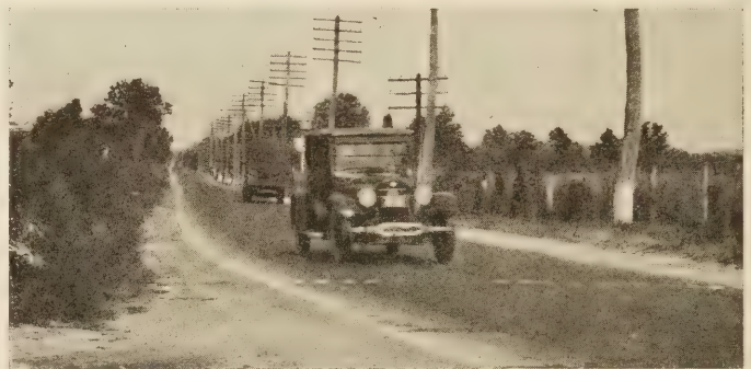
FIG. 10.—Test 19, made on a 24-foot bituminous macadam road at a 20° curve with a plane superelevated section and center line, shows a better separation of the traffic than test 16 (Fig. 9) made on a similar road with crowned superelevated section
